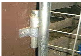
Wallpockets can be utilized to connect to walls.
